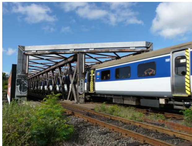
PARNELL RISE Overbridge: 2009: shown from road level with The Strand Hotel to the right, and from track level showing steel ties added in 1974
